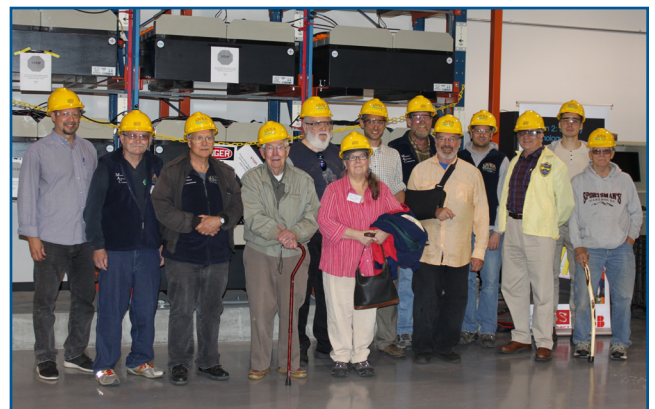
Above: During the summer of 2018, MAC members toured GVEA’s Battery Energy Storage System (BESS).
